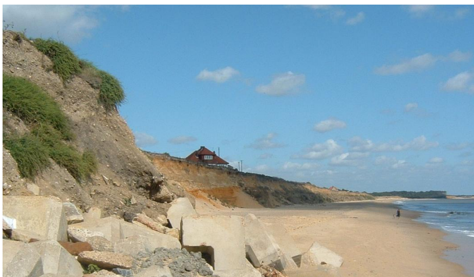
Fig. 4. Rapidly eroding soft rock cliffs along the Suffolk coast (close to Southwold) with residential properties only a few metres from the cliff edge. Photo courtesy of Dr Sally Brown.
