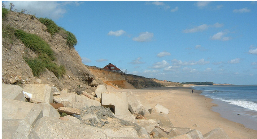
Fig. 4. Rapidly eroding soft rock cliffs along the Suffolk coast (close to Southwold) with residential properties only a few metres from the cliff edge. Photo courtesy of Dr. Sally Brown.
