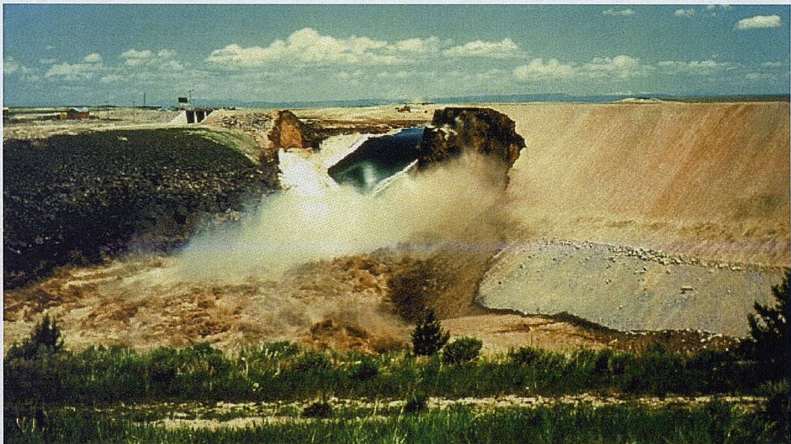
Figure 1.1b: Failure of Teton dam. Photo by Mrs. Eunice Olson, 5 June 1976. Arthur Gibbs Sylvester, University of California 2
