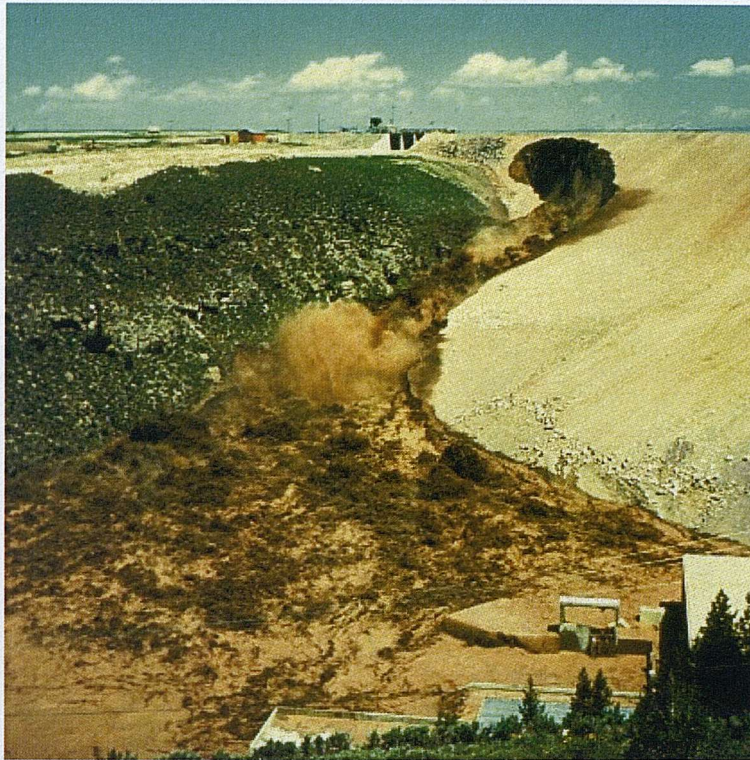
Figure 1.1a: Failure of Teton dam. Photo by Mrs. Eunice Olson, 5 June 1976. Arthur Gibbs Sylvester, University of California 2
