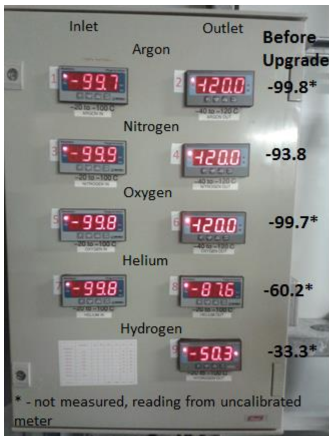
Figure 40 Picture showing dew point readings at the 1st stage purifiers after upgrade the purifiers.
