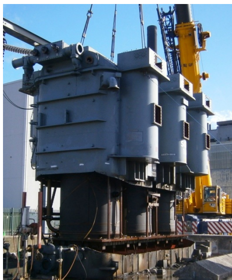
Figure 7 – Tank removal from a tri-phase 3-limb transformer in a coal-fired power station.
