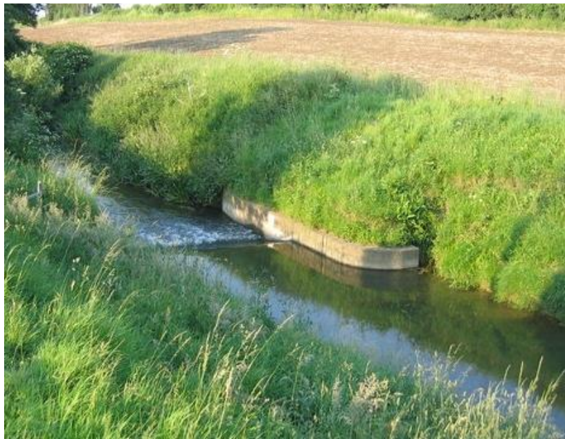
Figure 7.1 Small Crump weir on the River Isbourne (4.5 m wide, 0.5 m high channel walls implying head differences of < 500 mm). Copyright David Stowell and licensed for reuse under the Creative Commons Licence
