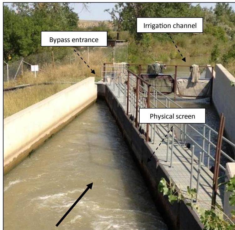
Figure 2.2 Example of a typical small-scale guidance facility for downstream moving fish, consisting of an angled physical screen to deflect fish away from a detrimental route (in this case an irrigation canal) towards a bypass channel (surface entrance). Solid arrow indicates direction of bulk flow.
