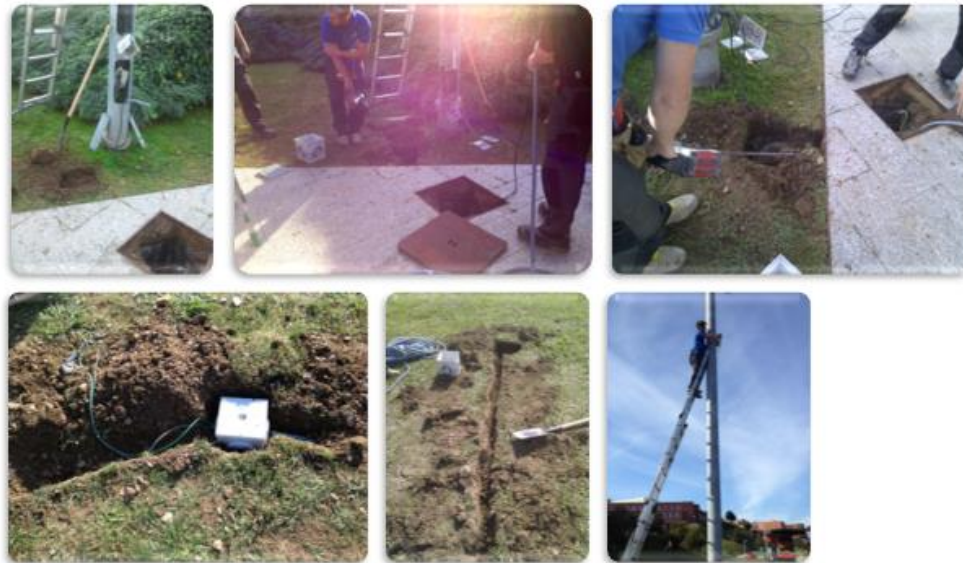
Figure 9. Soil moisture sensors installation in parks and gardens
