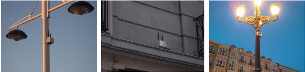
Figure 4. Examples of repeaters installation
