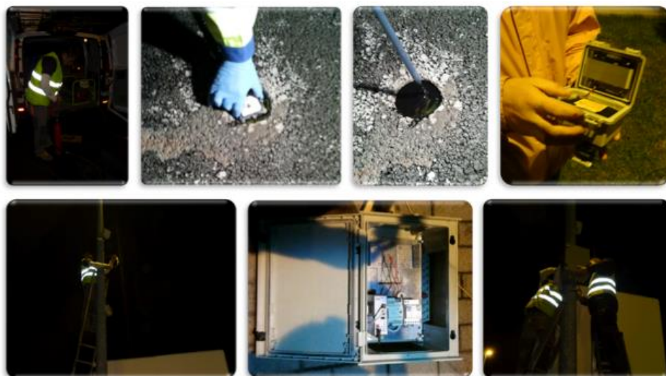
Figure 7. Traffic sensors installation in the main roads of the city
