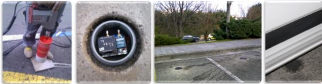
Figure 6. Examples of parking sensors installation
