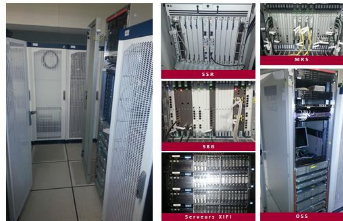
Figure 30. 4G/IMS installation (2)
