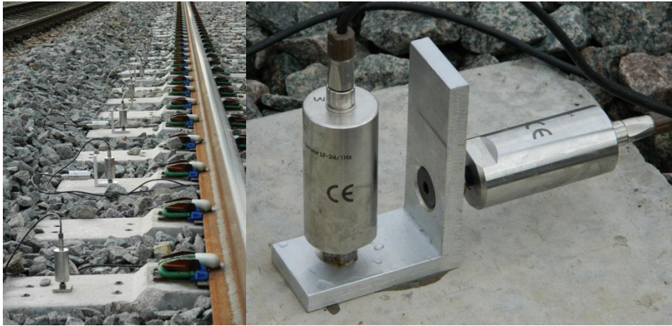
Figure 7. (a) Geophones on the sleeper ends, (b) oriented to measure vertical and lateral velocities
