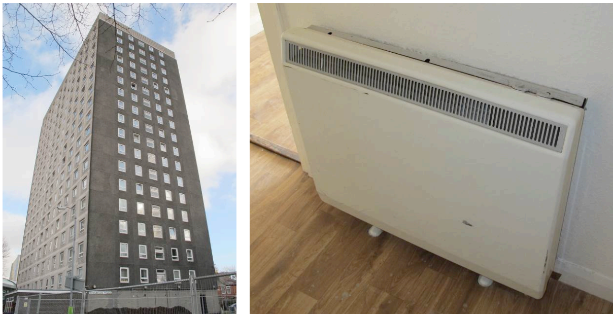
Figure 1. One of the two identical 17-storey tower blocks (left) and a storage heater in one of the flats (right).
