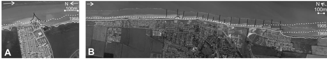
Set-back adjacent to 140m of shore parallel rock armouring and groynes constructed since 1978.
