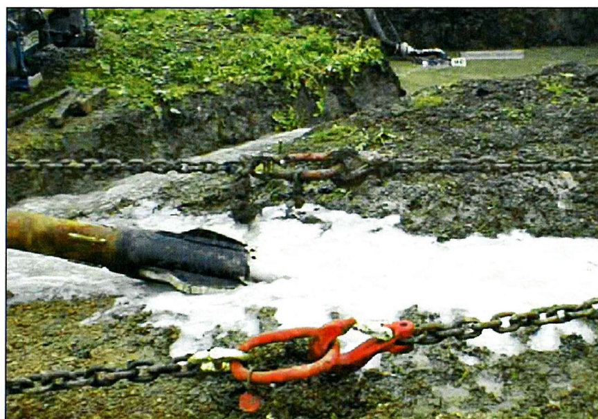
Figure 4.20 Overwash bit about to pierce the ground surface, drilling fluids being pumped into the annulus between overwash casing and drill rods.
