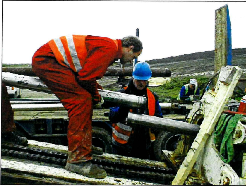
Figure 4.29 Connecting screen sections by hand, applying grease to prevent galling.
