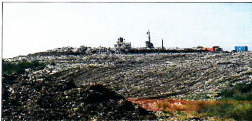
Figure 3.9 Tipping in layers. The most recent layer advances across the phase [Rainham, 1998].
