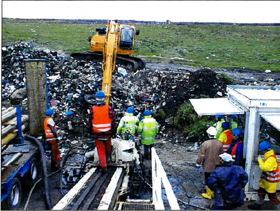
Figure 4.33 Everyone waits as the waste is excavated to find the end of the well screen.
