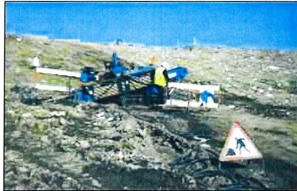
Figure 4.1 Mini-rig at Rainham for trial drilling.
