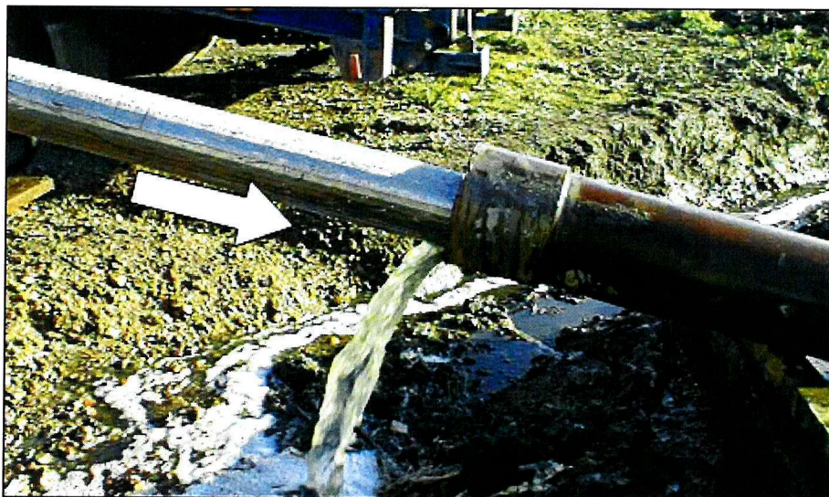
Figure 4.30 Well screen being pushed into overwash casing after drill rods were removed.
