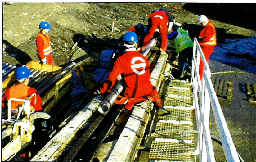
Figure 4.28 Adding a new length of well screen. Remaining lengths of screen in crate on left.
