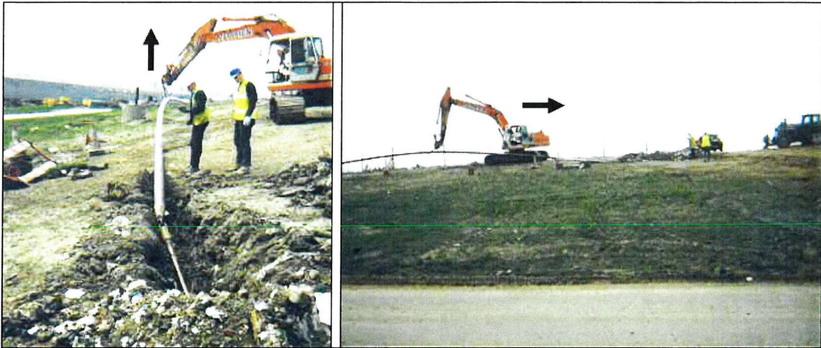
Figure 4.4 a) Excavator lifts well screen allowing it to pass into the exit trench at the correct angle, b) excavator feeds screen into the borehole to assist the pulling action of the rig.
