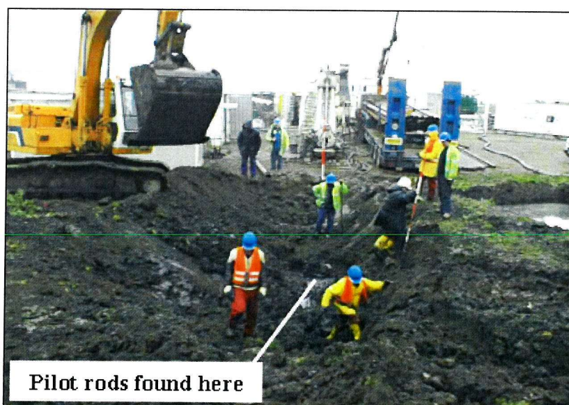
Figure 4.21 A 2m deep pit was excavated to find the end of the drill rods which had moved during overwashing.
