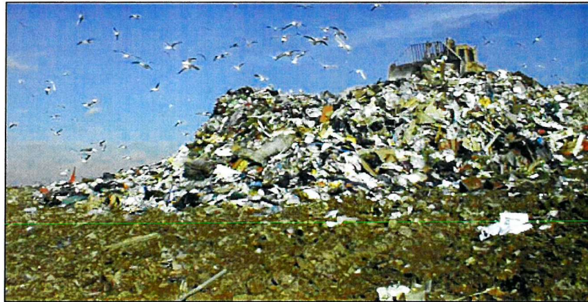
Figure 3.10 The tipping face is advanced over the previous layer of daily cover [Rainham, 2000].
