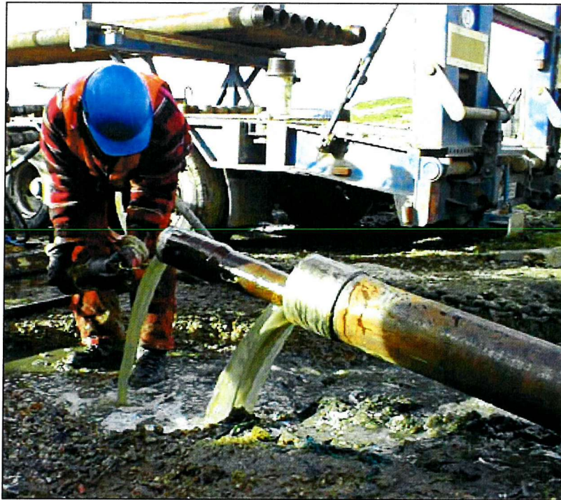
Figure 4.25 Drilling fluids and leachate flowing from overwash casing and drill rods.
