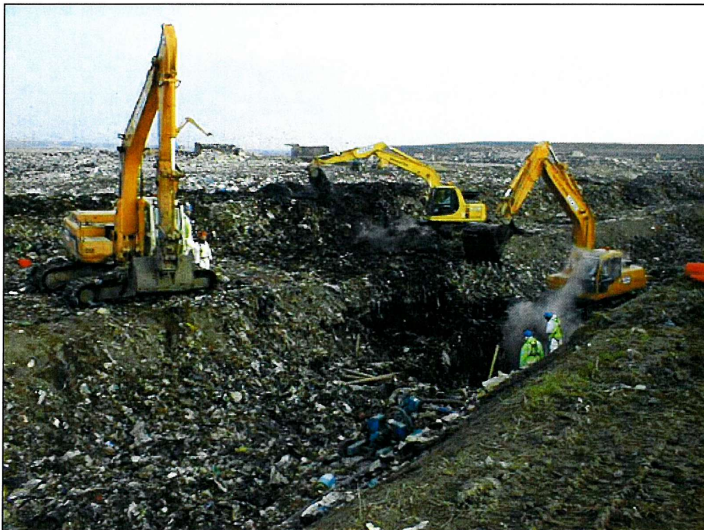
Figure 1.4 Excavation of trench in waste for installation of drainage system [Rainham Phase 1, Jan 2001].
