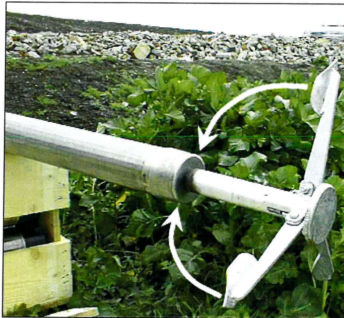
Figure 4.27 Sprung anchor fitted to leading end of well screen to fix it in the waste. Leaves are folded in direction of arrows as it is pushed through the overwash casing.
