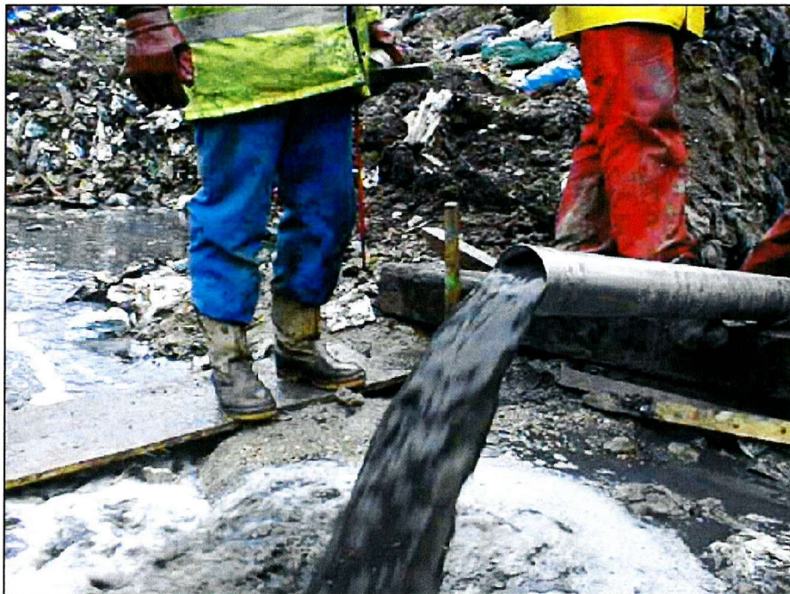
Figure 4.34 Leachate flowing from HW1 after the cap was removed.
