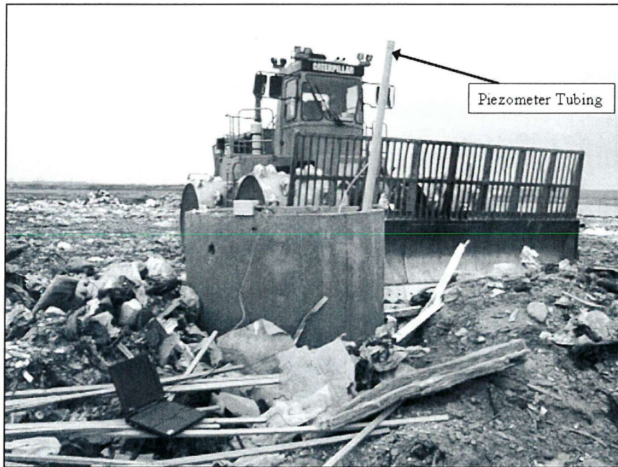
Figure 2.1 Large plant must work around vertical wells (and piezometers) and collisions are common. Here the piezometer tubing is protected by a concrete ring [Rainham 1999].
