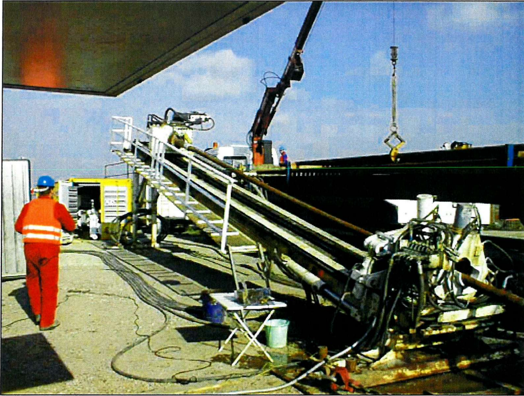
Figure 4.16 1000kN pullback capacity drilling rig at HW3.
