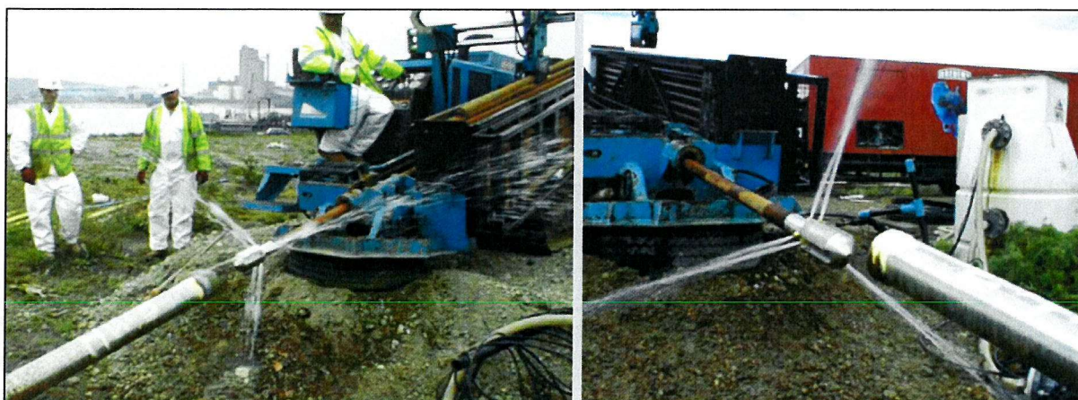
Figure 6.1 Small directional drilling rig used for well development, showing jetting head in action.
