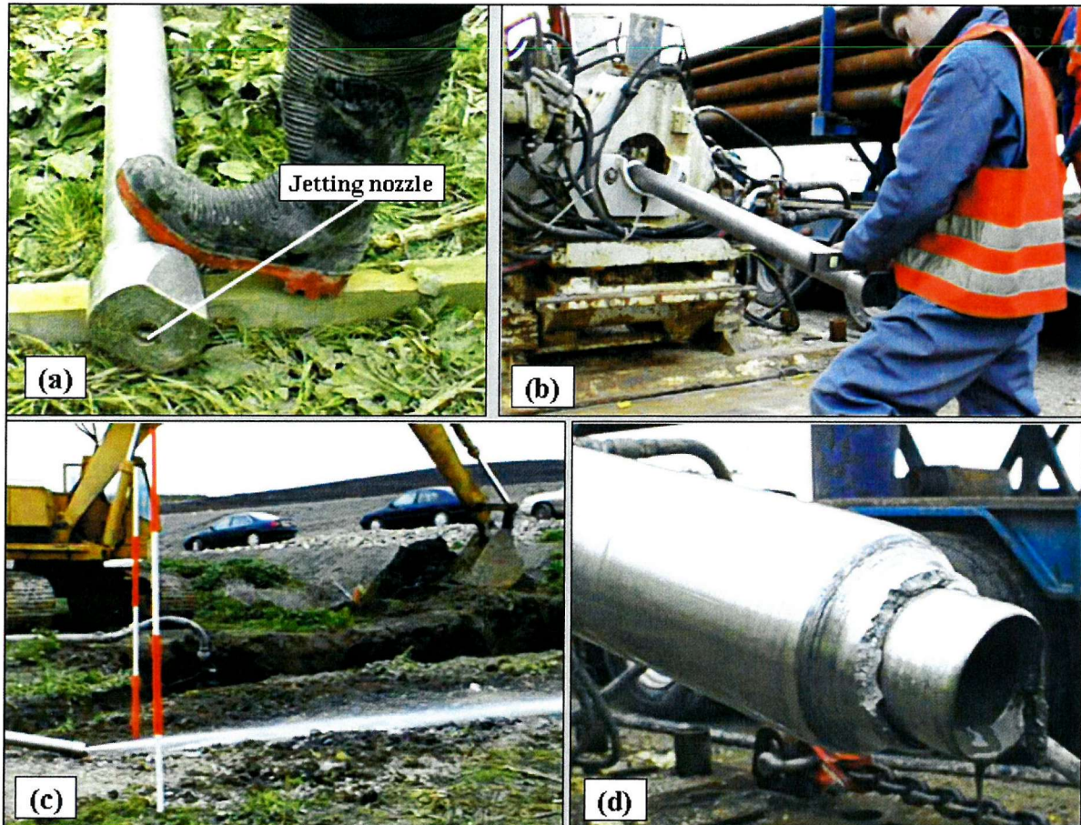
Figure 4.17 (a) Blunt-end drill bit with jetting nozzle, (b) aligning drill bit for guidance system, (c) jetting at start of pilot borehole, also range-rods for TruTracker, (d) blunt-end of drill bit sheared off.
