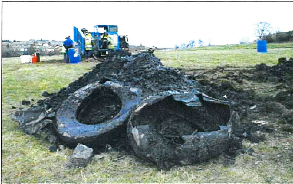
Figure 4.53 Lorry tyres that had caused the obstruction during pre-reaming, note how they have been ripped by the action of the aggressive reamer.
