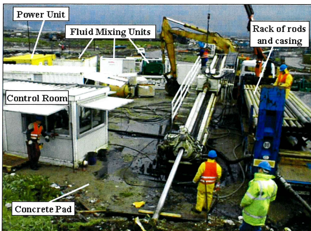
Figure 4.15 Site set up for installation of HW1.
