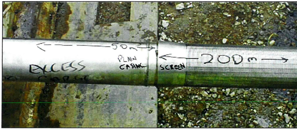
Figure 4.31 200m of 1mm slot width screen were installed to the far end of the borehole followed by 50m of plain casing to the surface.
