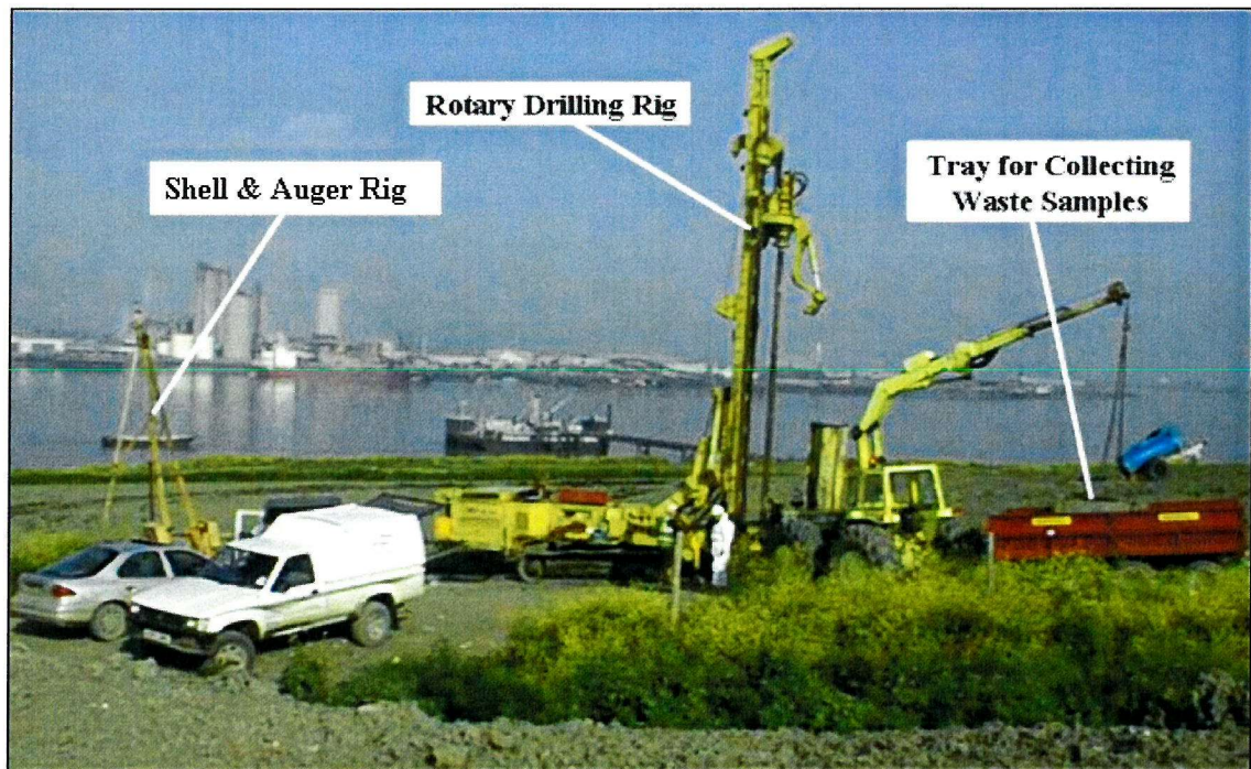
Figure 5.3 Two rig set-up for installing piezometers. Rotary rig to drill borehole, shell & auger rig to clean out temporary casing and complete installation [Rainham, 2000].
