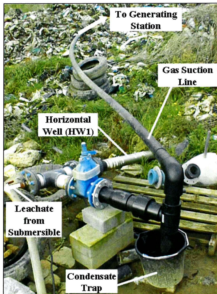
Figure 5.19 Gas Extraction Connections at HW1
