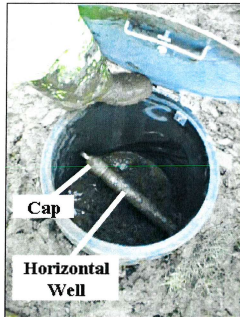
Figure 4.57 Capped end of completed horizontal well, with inspection cover.
