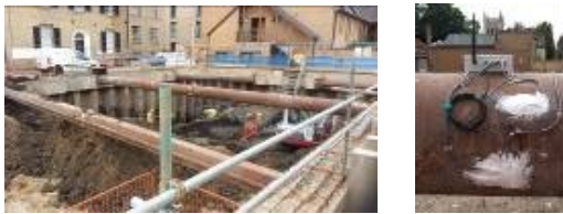
Figure 7. Field deployment of the wireless strain sensor network at the Trinity Hall excavation site.
