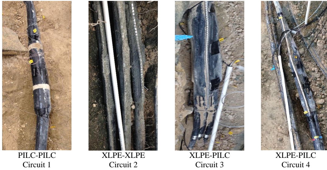
Fig. 64 Cable joints under investigation
