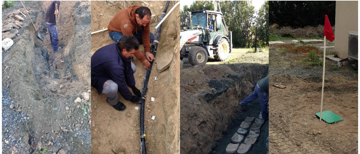
Fig. 66 Excavation of cable joint, installation of TCs and cover of cable joint.
