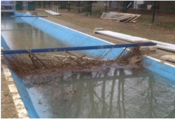
Fig 3: 0.45 m high wooden dam
