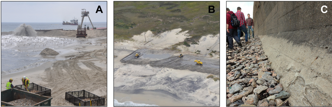
Figure 1. Three examples of typical coastal hazard mitigation practices: (A) beach replenishment in Monmouth, New Jersey (USA), nine months after Hurricane Sandy (photo: A. Coburn, Program for the Study of Developed Shorelines, http://www.psdw-wcu.org/ ); (B) artificial dune reconstruction following an overwash event on Highway 12, North Carolina Outer Banks (USA) (photo: A. Coburn, PSDS); and (C) concrete seawall on the Channel Island of Jersey – note the pitting and fresh scour (light gray band) along the wall base just above the shingle toe.
