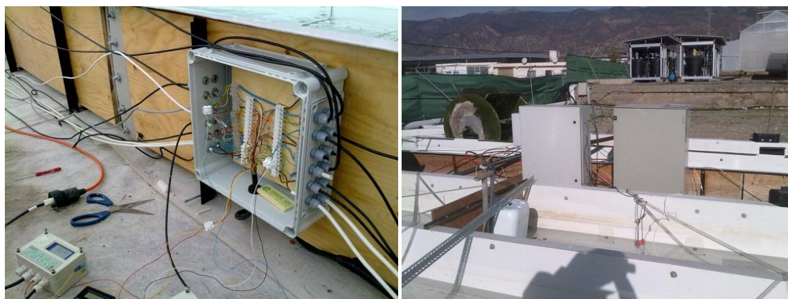
Figure 28.- Left: Detail of the connection box installed in the wall of one of the raceways where the 36 wires cable collected the electrical signals of probes to send it to the control room. Right: Cabinets where all the probes were connected to the transmitters to protect the electronic equipment
