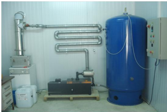
Figure 32.- Flue gas supply to the raceway. Left: flue gas production system with diesel boiler (white), gas compressor (black) and gas pressure vessel (blue). Right: sump view with flue gas bubbling in a microalgae culture.
