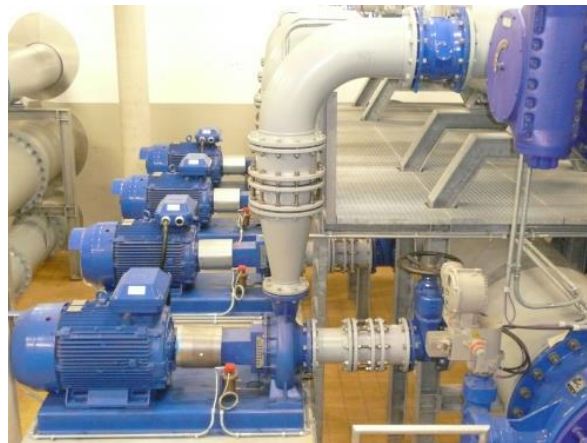
Figure 2.33: A typical instalation of PAT (Orchard 2009)
