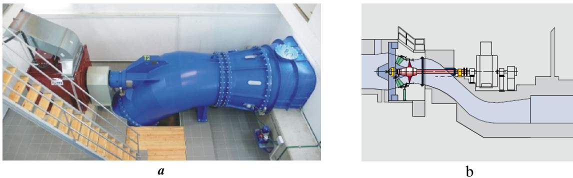
Figure 2.24: (a) An instalation of the S type Kaplan Turbine (Chongqing Hydropower Equipment Co. 2016) (b)cross section of an S-turbine and generator(voith hydro 2016)
