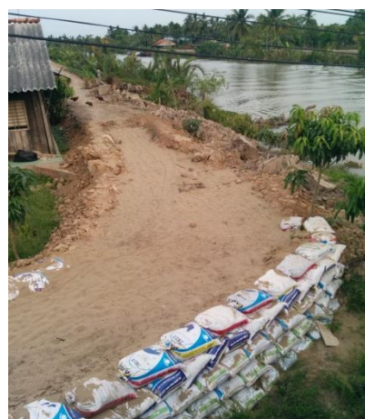
Image 4.1: A high river dyke in the final stages of construction
