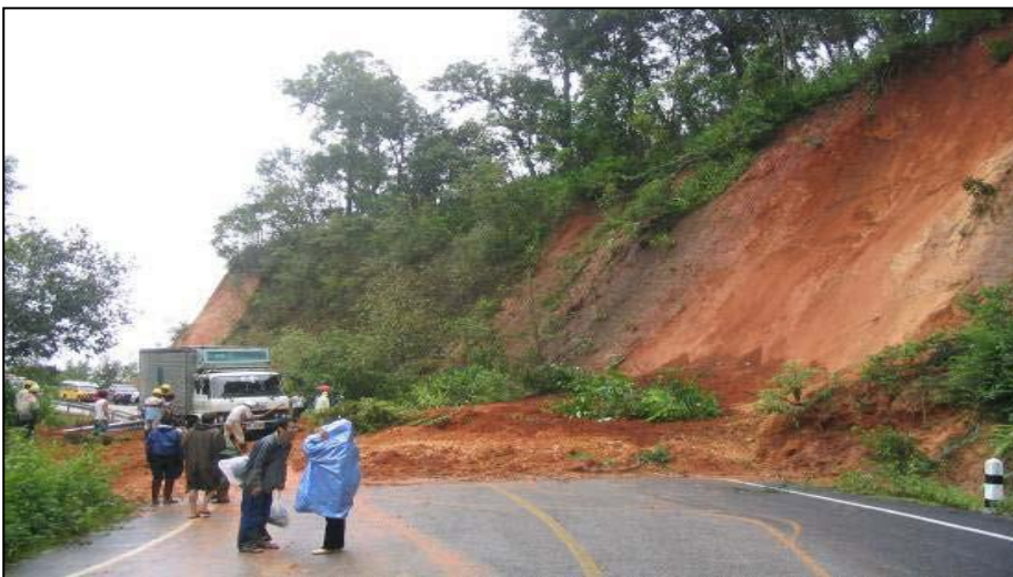
Figure 2.14 Road side cutting failure at Mae Fa Luang district, Chiang Rai province (DMR, 2011b)
