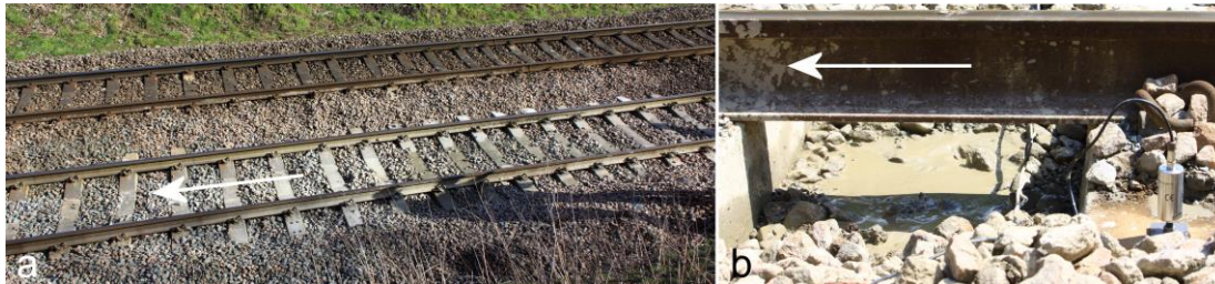
Figure 2: (a) Wet bed prior to track renewal. (b) Close-up of worst region – slurry and pea gravel also visible. Arrows show direction of travel on affected line.
