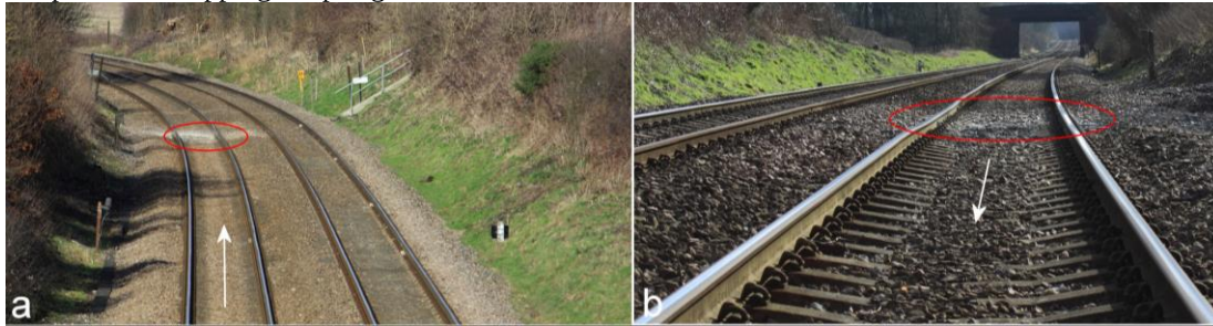
Figure 1: (a) View from bridge in the direction of travel (left line). (b) View from beyond the wet bed area looking back towards the bridge. The wet bed area is circled. Arrows indicate the direction of travel on the affected line.
