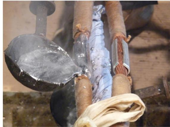
**Figure 1.** Photograph showing the application of molten solder to a ferrule in a straight lead joint, used with permission from [9].
