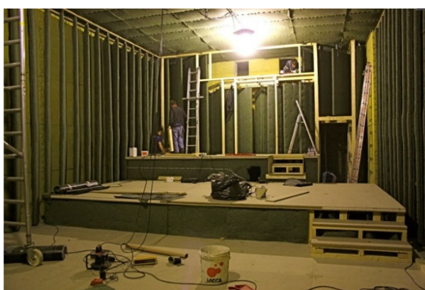
Figure 8: Detail of acoustic treatment of the walls. Behind the waveguides are multiple-membrane absorbers
