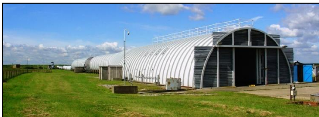
Figure 1. The air blast tunnel (ABT) at MoD Shoeburyness, UK [1].
