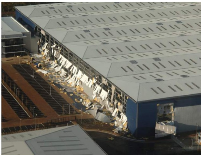
Figure 2.4.7: Outward Displacement of Cladding on Back Wall of Warehouse (Atkinson, 2011a)
