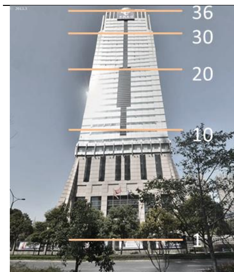
Figure 5.7. Estimation of the error in the building height measurement of a skyscraper with an office use in Hangzhou, China. Image sources as referenced in figure labels.
