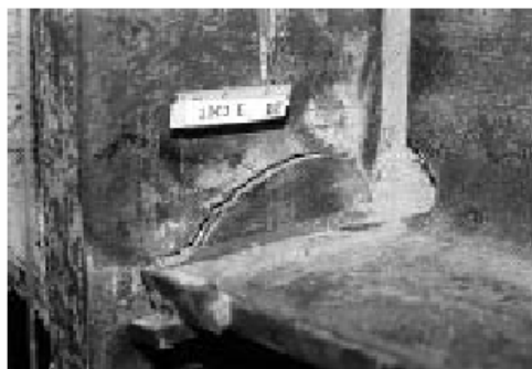
(c) Column flange "divot" fracture
