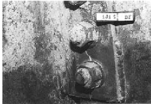
(f) Vertical fracture through beam shear plate connection
