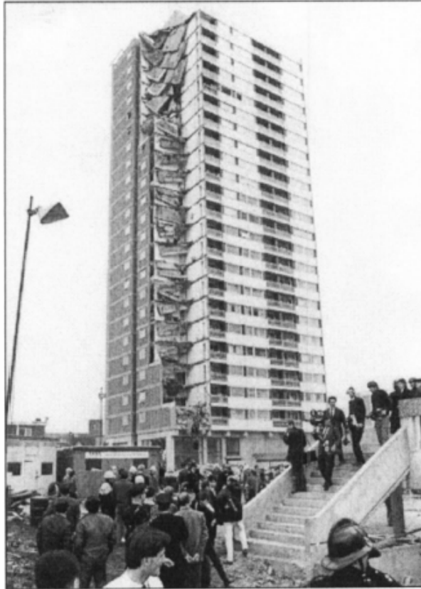
Fig. 2.1. Ronan Point after collapse (Pearson and Delatte 2005)
