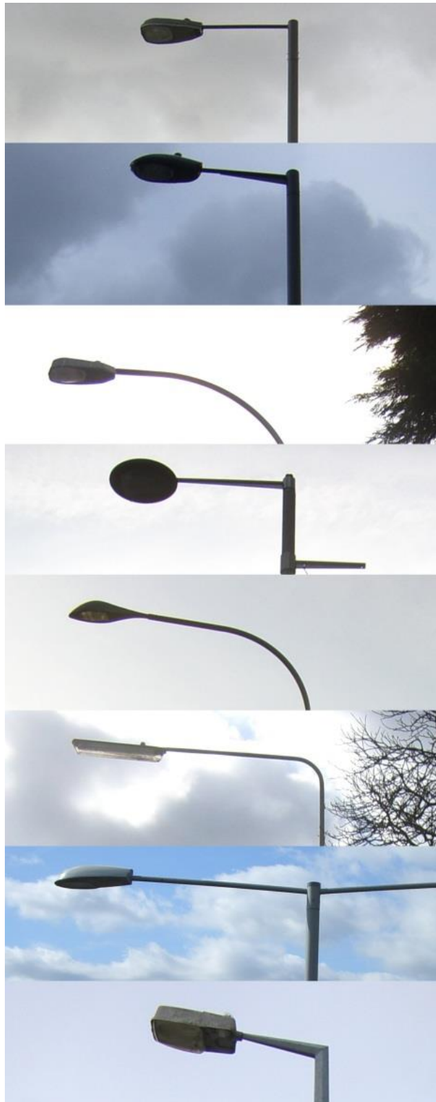
Figure 3.1 - Various lighting columns with assorted projection brackets.
