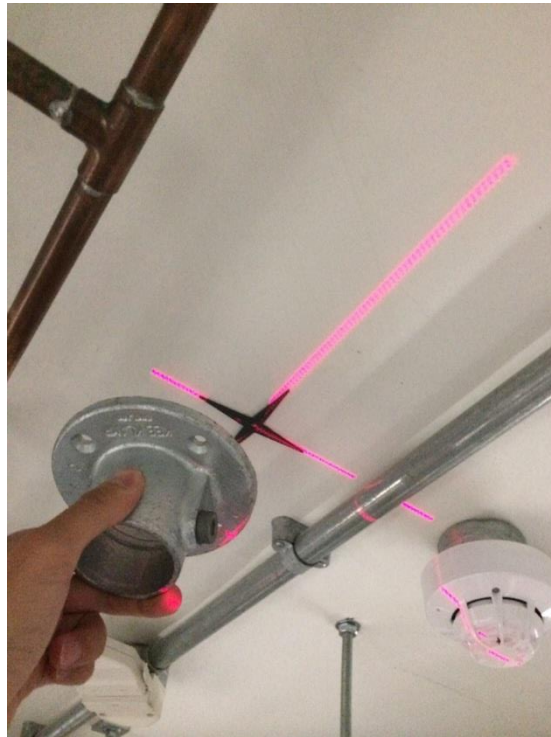
Figure 4.17 - Drill calibration tool which allowed the markings for where the holes needed to be made for the flanged ceiling mount.
