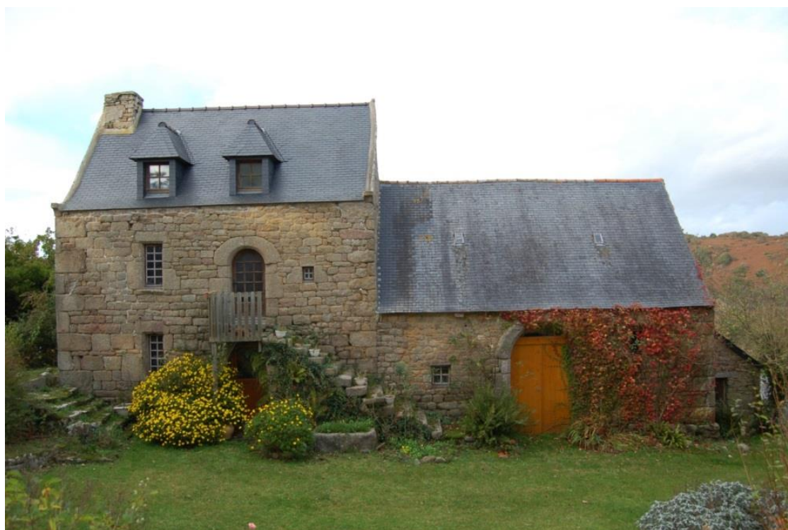
Figure 57 – One of the many buildings on the headland of le Yaudet constructed from the local granit de Plouaret . The roughly squared nature of the masonry is similar to the construction used in the intertidal structures throughout the estuary.
