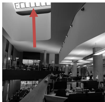
Figure 3: The atrium and the roof top dampers
