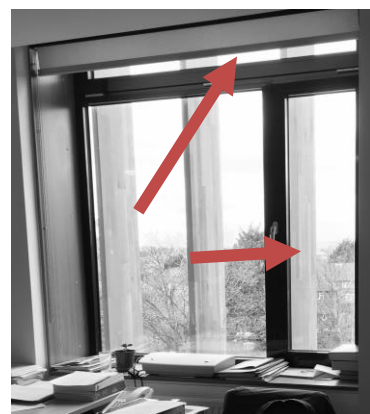
Figure 5: Levels 4 and 6 windows and hoppers
