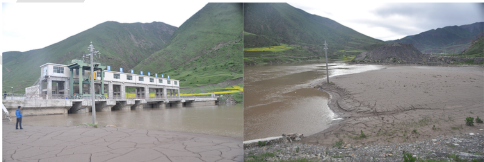
Fig. 5. Extensive sediment deposition in the reservoir of the Jiqian SHP plant in Biru County.
