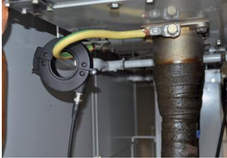
Figure 2.3.2 A RFCT sensor installed on the earth conductor of single-core cables [58]
