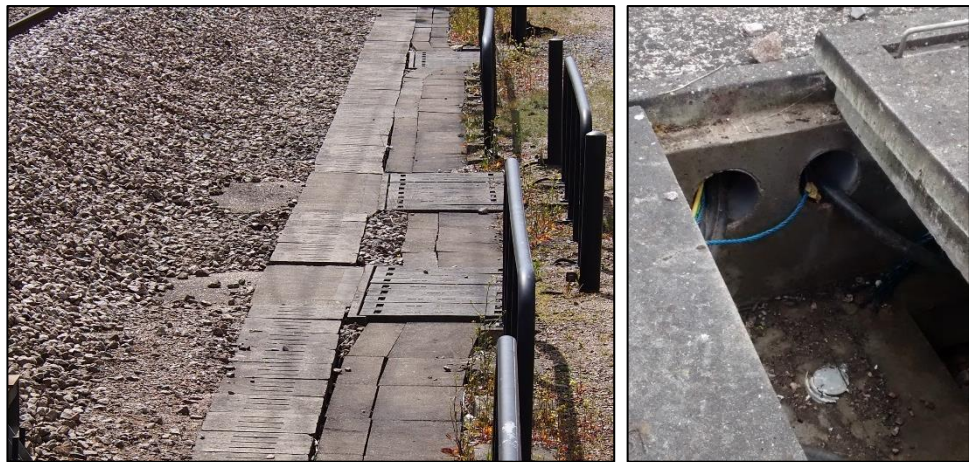
Figure 3.11 (a) surface view of UTX and inspection chambers next to the ballast shoulder, (b) view inside UTX inspection chamber.
