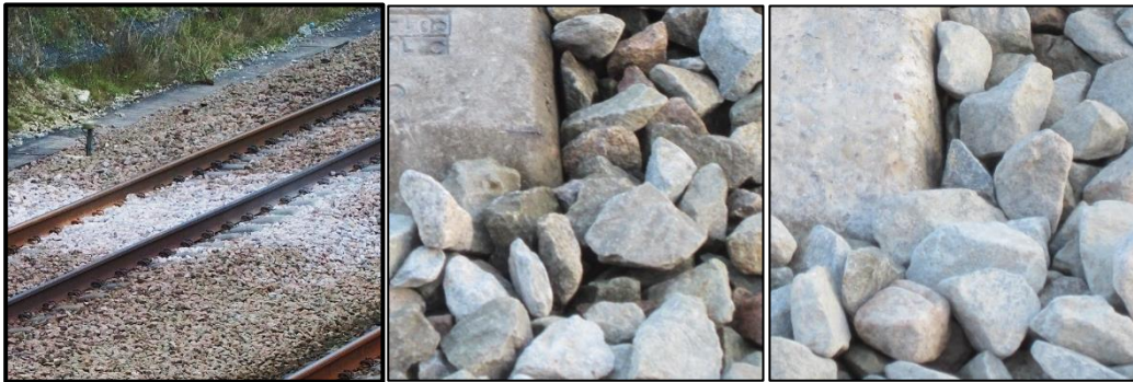
Figure 9.20 (a) A defect zone, (b) ballast and sleeper end outside a defect zone and (c) inside a defect zone.
