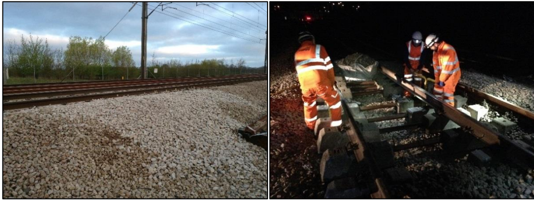
Figure 9.34 Photographs of installing new sleepers with USPs.
