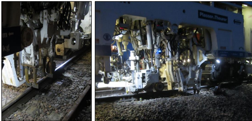
Figure 2.8 Photograph of tamping machine (a) tines above ballast (b) in operation.
