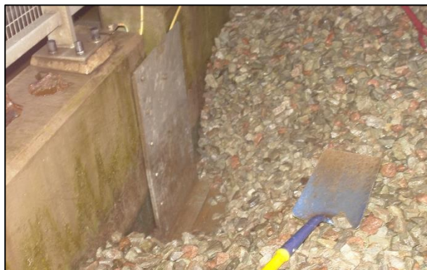
Figure 3.13 Photograph of expansion joint plate at Rainham.
