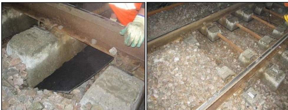
Figure 9.33 Photographs of retrofitting USPs to sleepers in situ.
