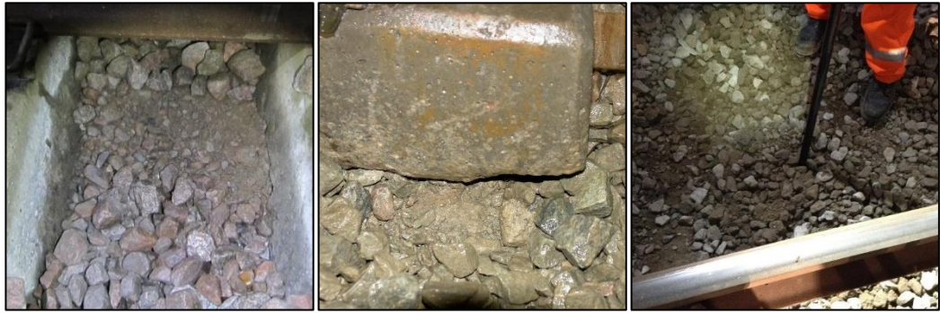
Figure 9.21 (a) Excavation into the ballast crib, (b) damage to sleepers, (c) track bed below sleeper level.
