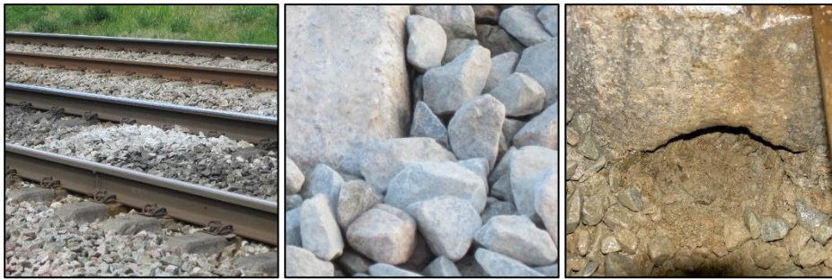
Figure 1.1(a) Visible track defect; (b) ballast abrasion; (c) damage to sleepers and ballast.
