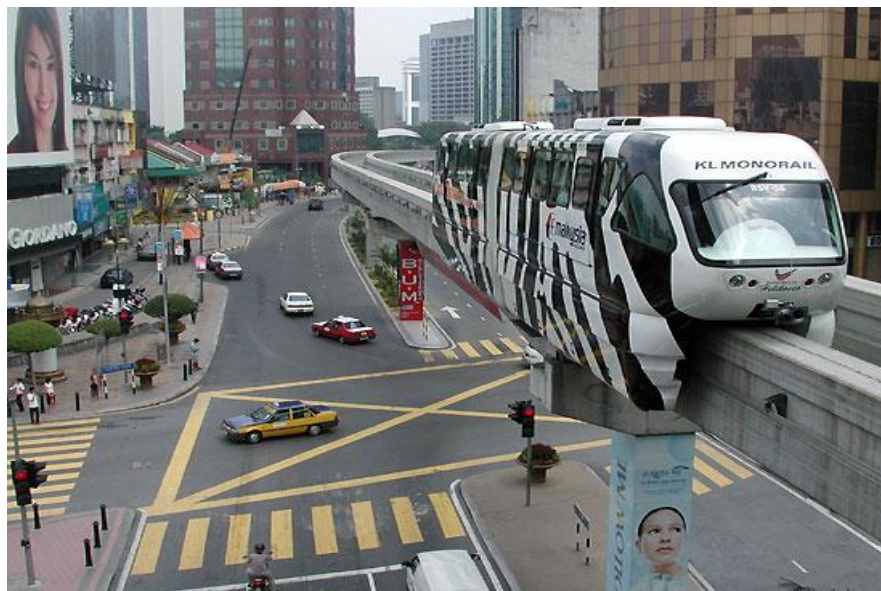
Figure 4.40 Looking north from Bukit Bintang Station. Unlike the monorails of Japan, long spans are not made of steel. Note the long distance between these two pylons over this intersection span.
