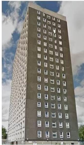
Exterior view of Tower A
