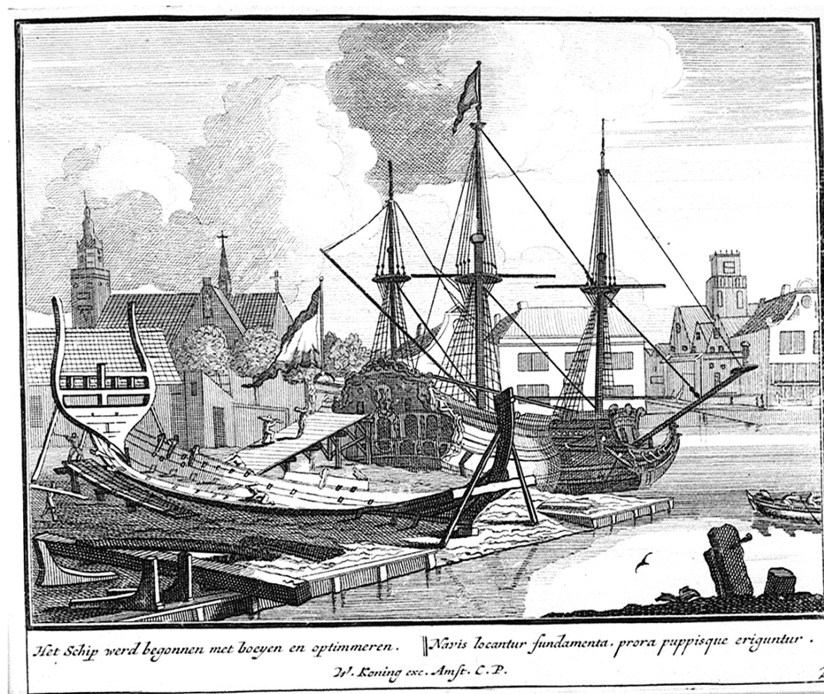
Figure 11 Dutch ship being built in the bottom based tradition. Planks are being fixed to each other by small cleats. (Image from a series of 16 engravings by artist Willem Koning at the National Maritime Museum. http://212.219.145.45/collections/objects/111178.html )
