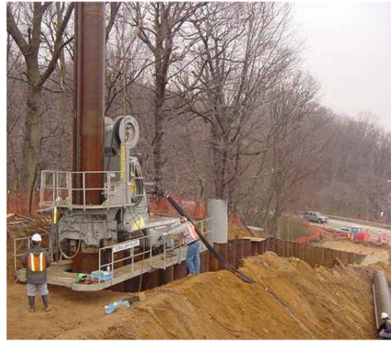
b) The installation of a wall of interlocking steel tubular piles near New York
