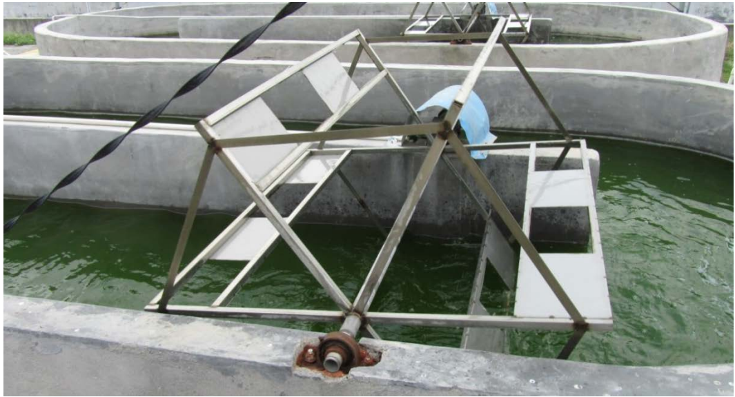
Figure 3.33. Part blade design from a 260 m 2 raceway located in Guangzhou Institute of Energy Conversion, Guangdong province, China.
