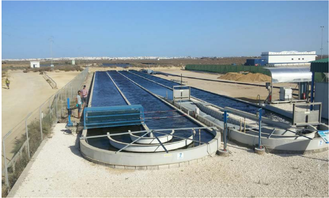
Figure 5.38. The 500 m 2 prototype raceway reactor located in Chiclana de la Frontera.
