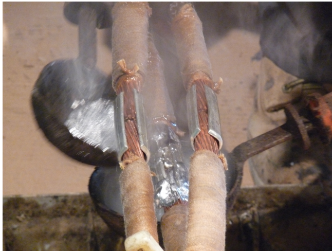
FIGURE 5.1: Photograph showing application of molten solder to the ferrules, used with permission from [76].
