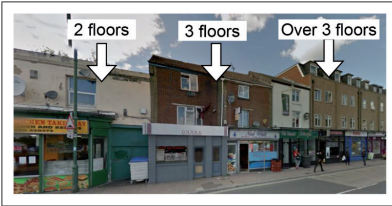
Figure 6. A row of terrace buildings that has varying floor counts. Address: Onslow Road, Southampton, SO14 0JD.
