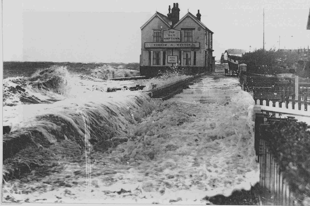
Plate 2.2. Wave Overtopping of Coastal Defences at Whitstable, 1949.
