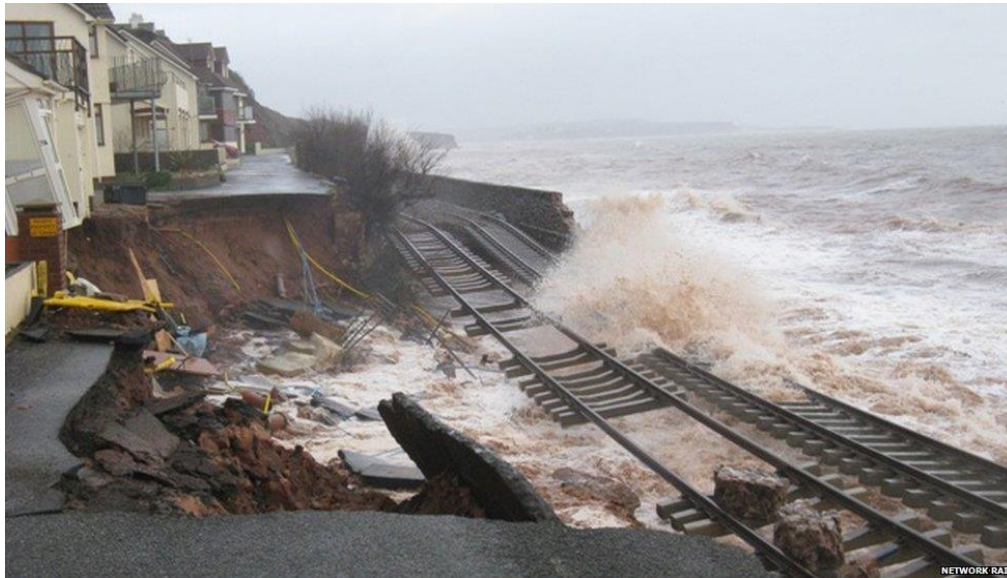
Figure 1.1.3 Wave impact damage sustained on the south coast of Devon during storm events in 2014, (NCE, 2014).
