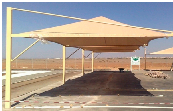
Figure 3. Image of existing car parking canopies.
