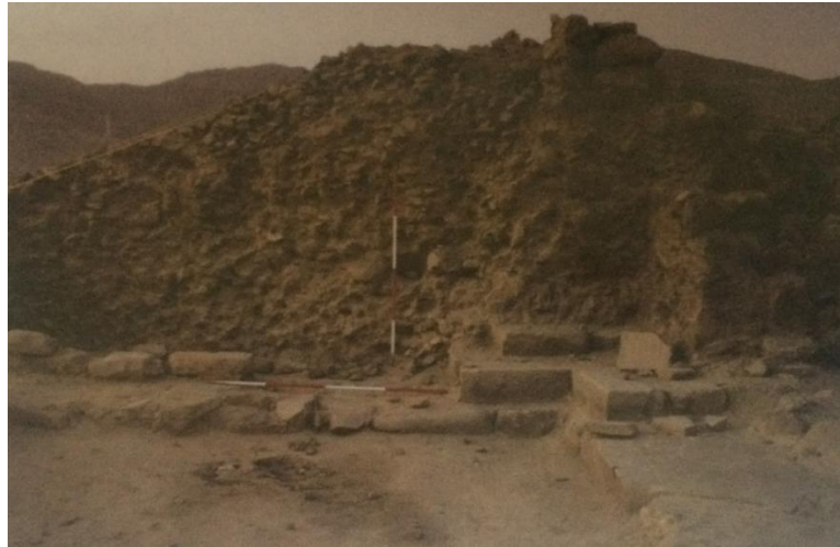
Figure 2.38.B: Debris that covered wall in north eastern side (Al-Sabail et al., 2006)
