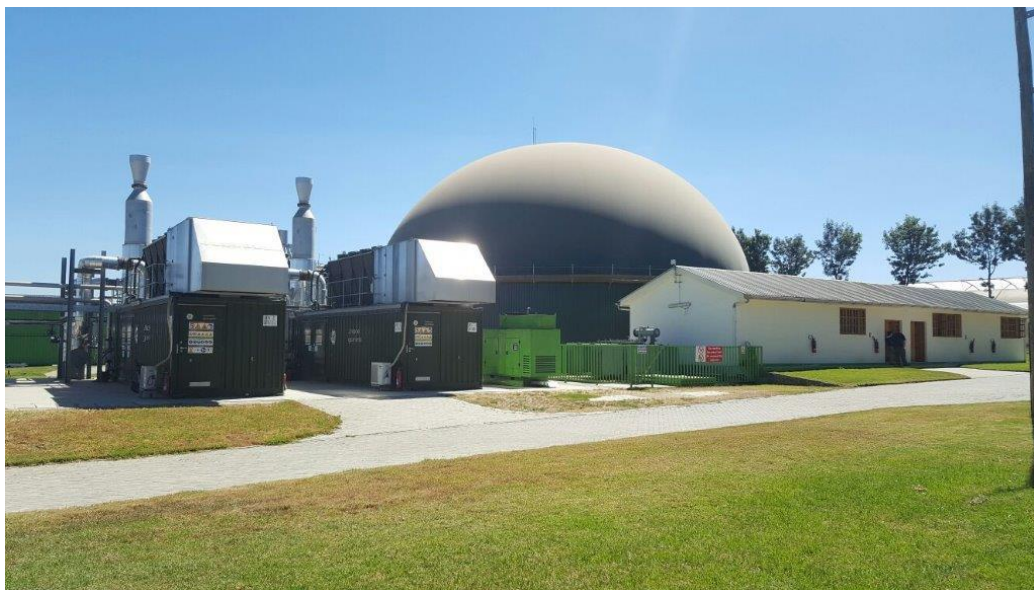
(b) View of the biogas plant showing CHP units (front left) and main digester (back right) (Photo courtesy of Ms Angela Bywater)
