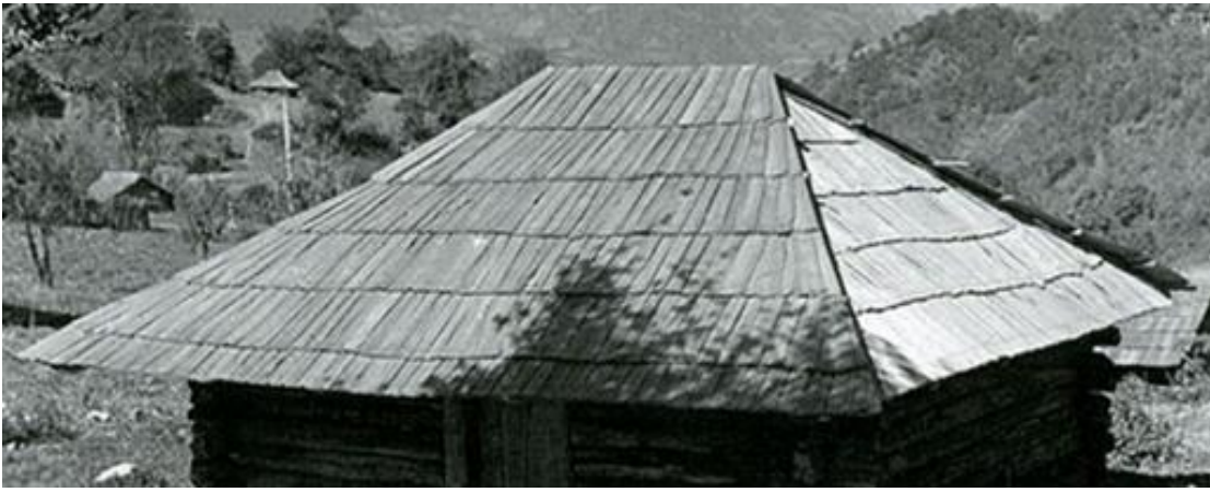
Figure 4.43. A classic example of the pre-Hispanic wood cutting technique called Tejamanil ( https://www.haikudeck.com/vernacular-architecture-art-and-design-presentation-kXq2yYOekp )
