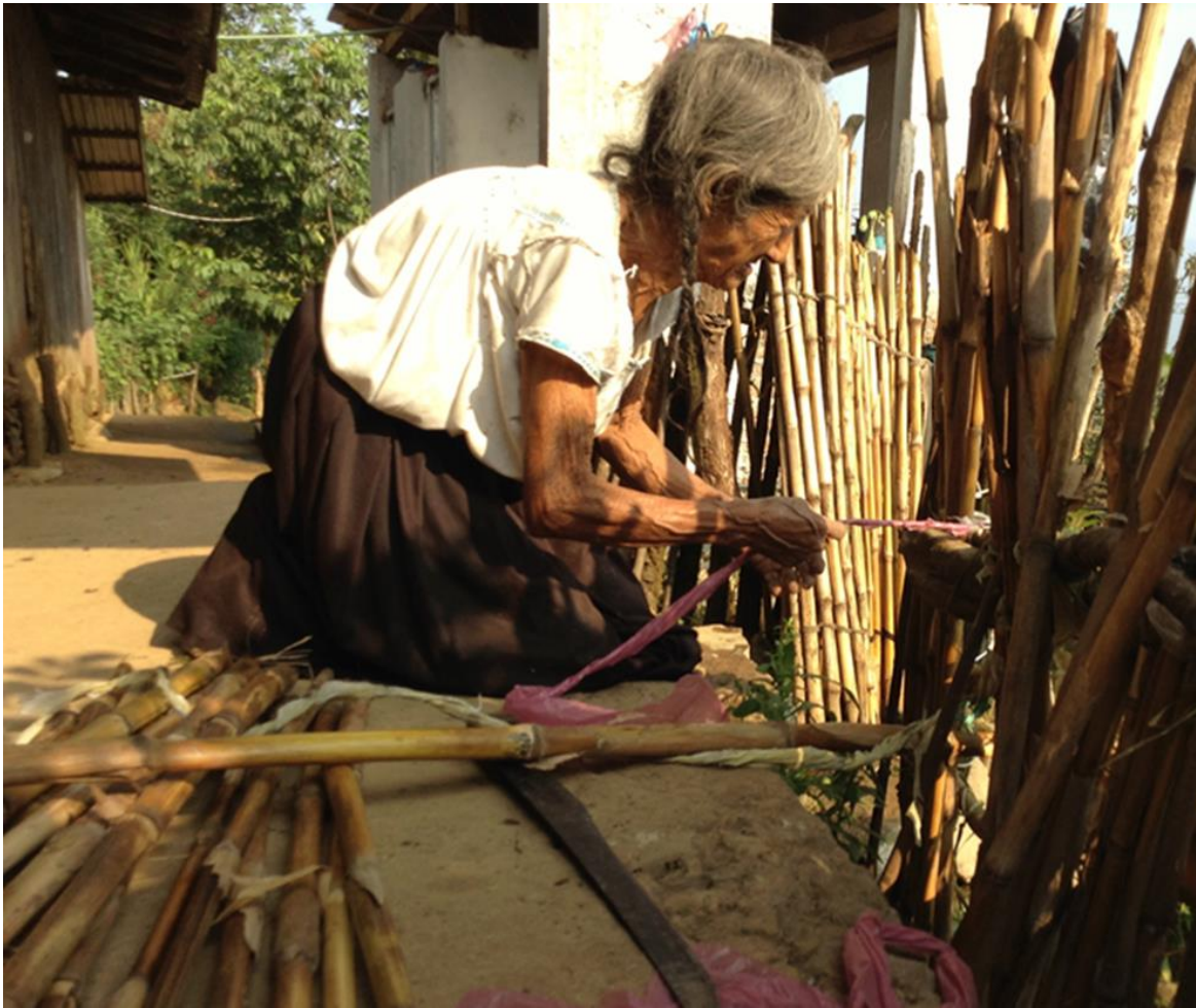
Figure 4.20. Dona Maria Antonia, showing us how to tie the thin sticks as they used to build the walls of the house. Now they use it sometimes to build fences, however in the past they used to do this for the walls, and instead of plastic bags they used the maguey fibres.
