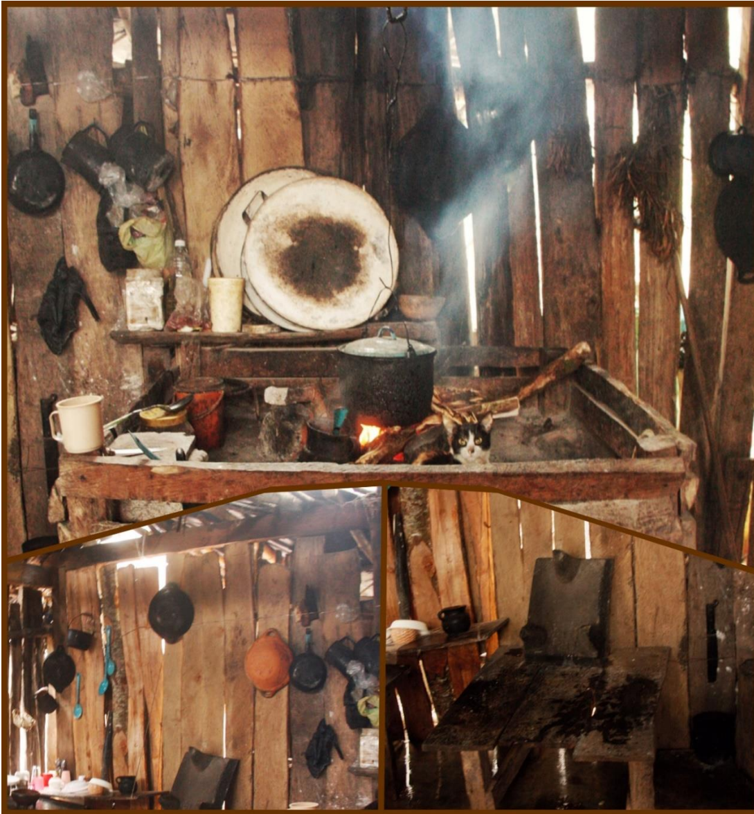
Figure 4.10. The brasero (lifted stove) is made with wood, big rocks in the bottom then sand all the way to the top. However, the fire place is made in the same way that they produced it in the past, with three stones to support the pots and pans “the only difference is that now we cook standing up, it is easier than our grandmothers used to work”.
