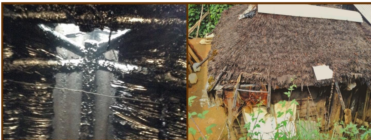
Figure 4.21. The kitchen from the above and the roof inside. The shape of the hip-roof is well represented in the photograph. Even if along the interviews people agreed that the grass was resistant enough, the perishable nature of the materials is evident. In Doña Rosa's house we could really see the weather damage and the lack of maintenance. Pictures taken by V. Quiahua
