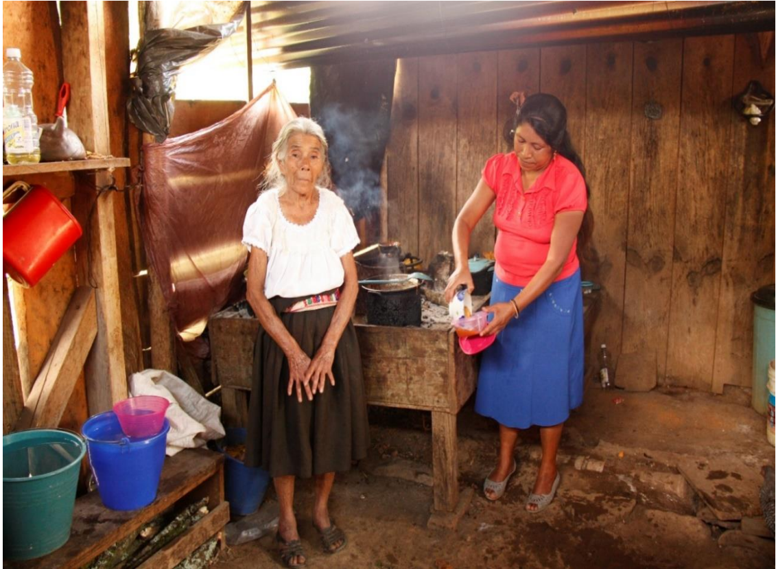
Figure 4.6. Eliazar kitchen is made with wooden cladding, nails, plastic bags and two pieces of corrugated metal sheets. The shape that the roof has is mono-pitched and the floor is the soil without materials. In the picture Eliazar is cooking and her aunt is warming herself near the fire
