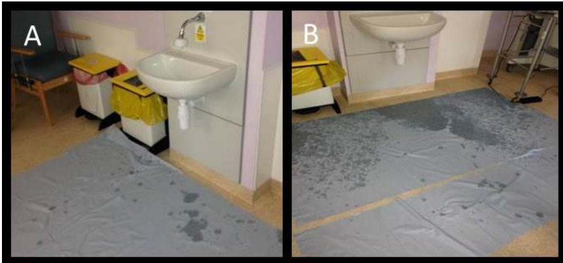
Figure 6.1 Effect of flow rate upon the dispersal of water droplets (splashing). Splashing is indicated by the darker patches on the absorbent material on the floor. A: tap with an outlet fitting (point of use filter) in place showing relatively limited splashing; B: the same tap with the outlet fitting removed showing a large amount of splashing onto the floor. Photos taken and provided by Jimmy Walker (Public Health England).
