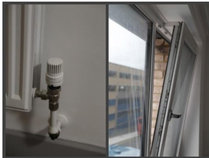
Figure 2 Indoor environmental controls available to Mayflower residents; radiator control valve (left), top opening tilt window with trickle vent (right)
