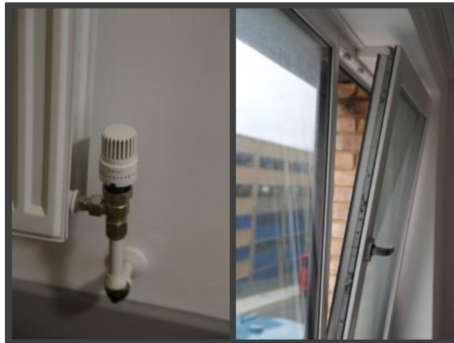
Figure 3.6 Photographs of indoor environmental controls available to Mayflower residents; thermostatic radiator control valve (left), top opening tilt window with trickle vent (right)
