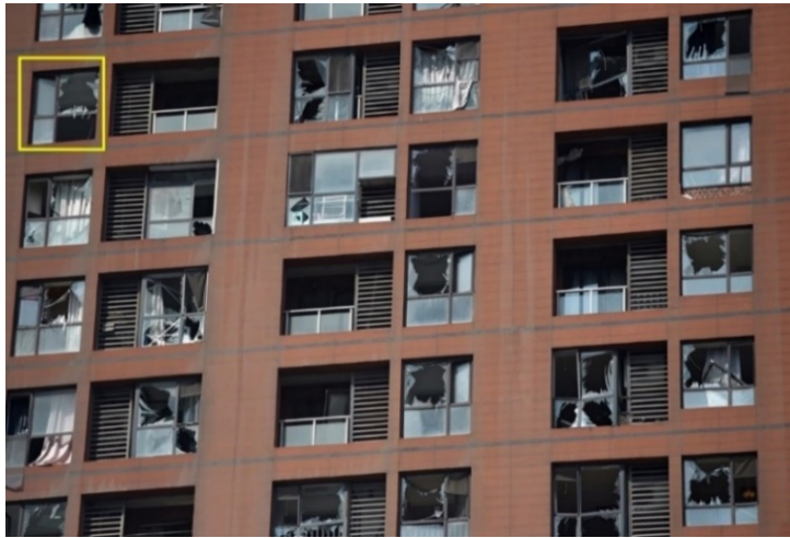
Figure 3.10: Windows damage near to the Tianjin explosion (BBC News, 2015).
