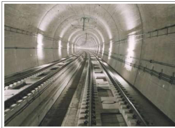
Figure 1.2: Slab track inside the tunnel at the Kyushu Shinkansen line (Yokoyama, 2000).
