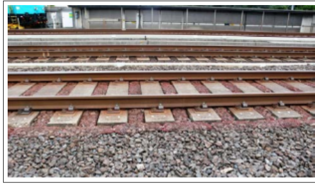
Figure 3.6: Ballast bags; the solution proposed in Japan (photo by T.C. Kao) (Jacobini et al., 2013).
