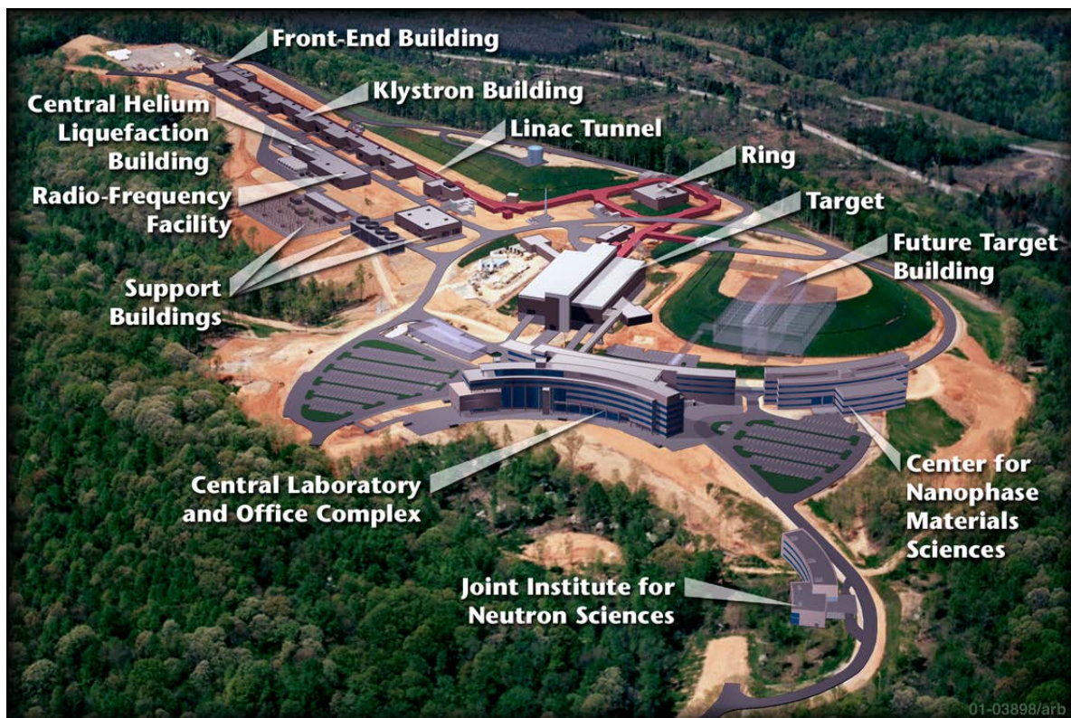
Figure 1. Schematic of the Spallation Neutron Source at Oak Ridge National Laboratory, Tennessee. The hydrogen ions for the linear accelerator are generated in the ‘front end’ building at the top left of the picture, and are accelerated down the linear accelerator (shown in red) to the ring, where protons are accumulated. During repeated circulation of the ring, more protons are added to ‘paint out’ the complete 200 m m x 70 m m elliptic proton beam. When this is complete (which occurs 60 times per second), the proton pulse is released into the ‘target’ building, the centre of which houses the sarcophagus in which the actual mercury target is housed. A possible future target building is shown in ghost outline (image courtesy of ORNL).
